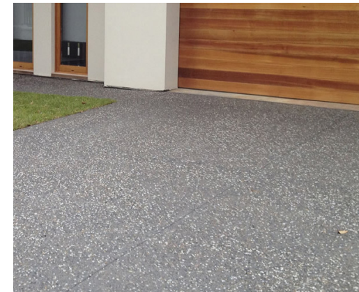
P4: Exposed Ag insitu-concrete (Podium)
